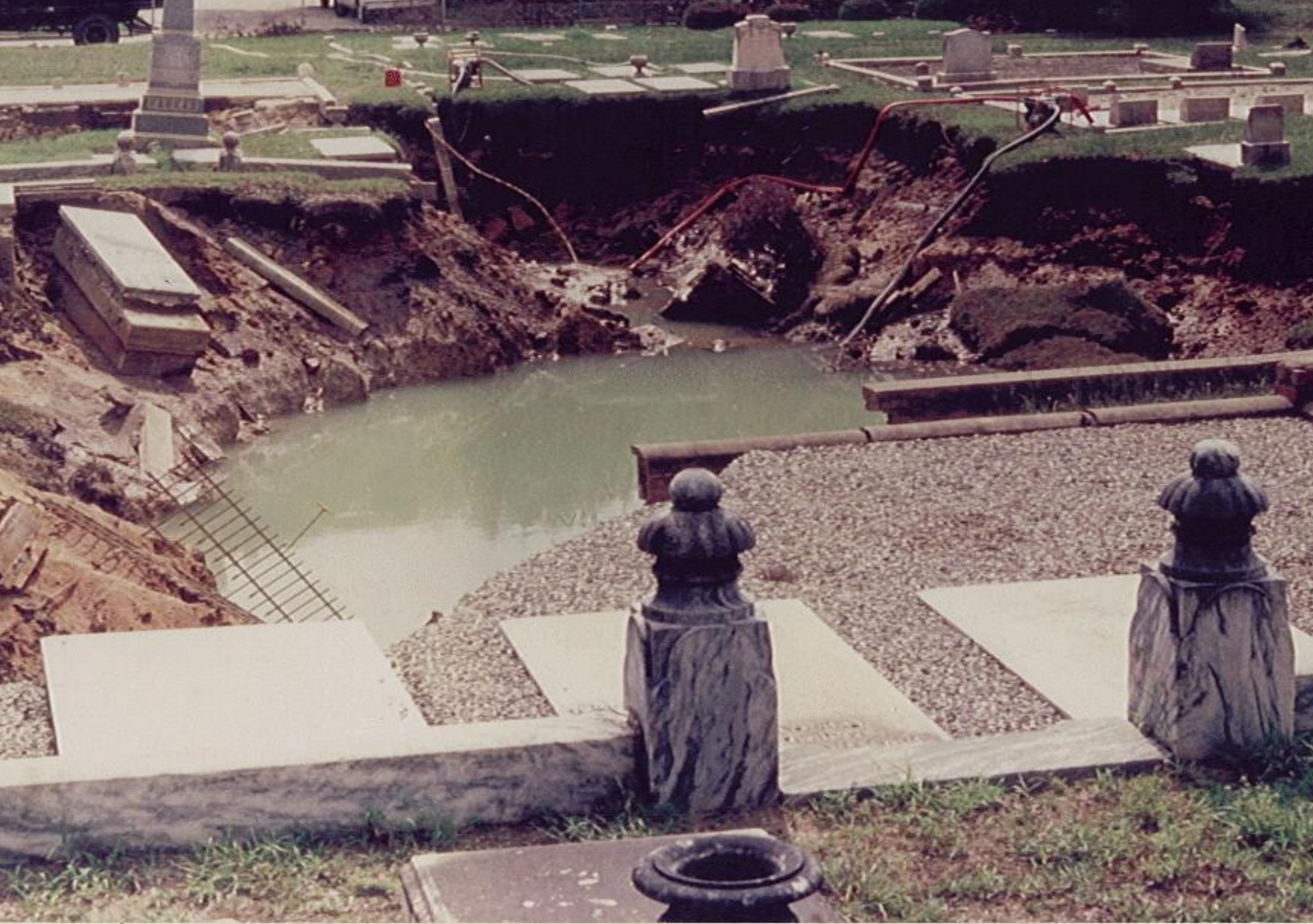
Sinkholes in Oakview Cemetery, Albany, Ga. - 7/94 by D.W. Hicks
